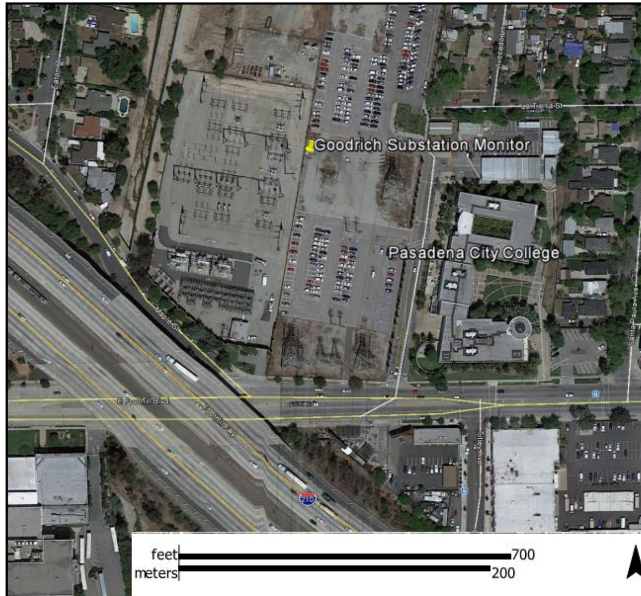
Figure 3-2 Goodrich Substation Noise Measurement Location
